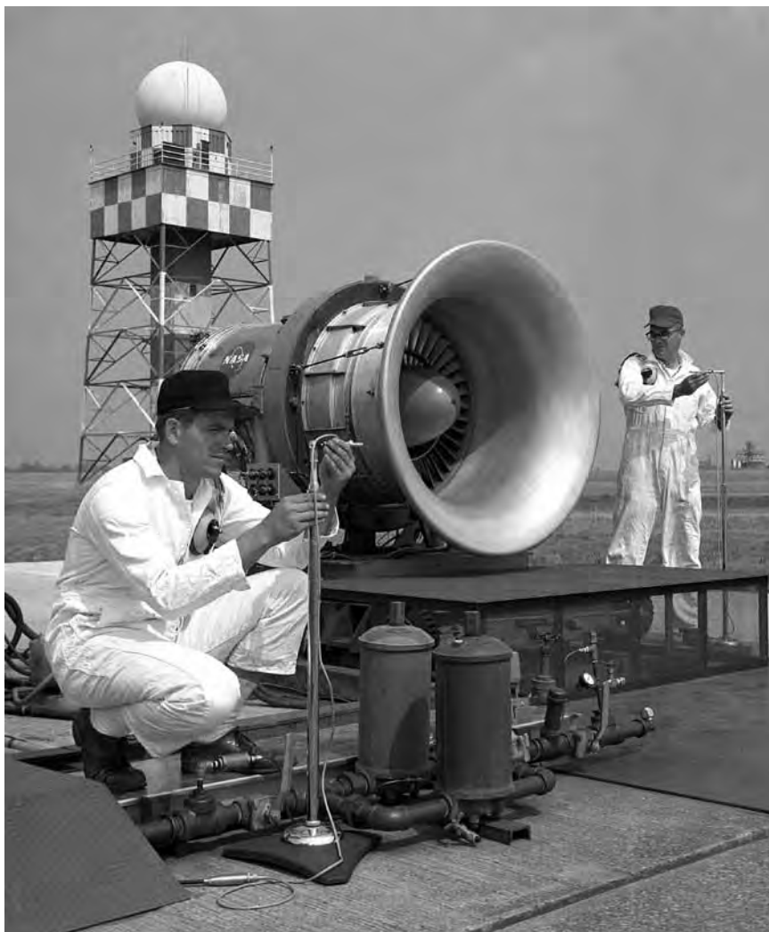
A jet engine is prepared for a test in 1967 as part of an early noise research program at Lewis Research Center. NASA.
