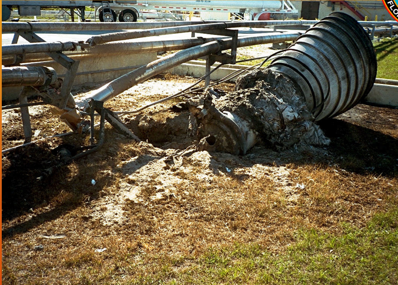
Main Engine Nozz-hole
