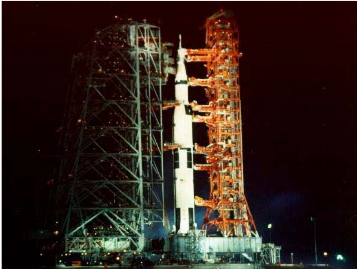
Removing the Service Tower, December 5, 1972
